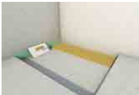
2. Preparation of the surface (flat surface), apply adhesive on the surface
