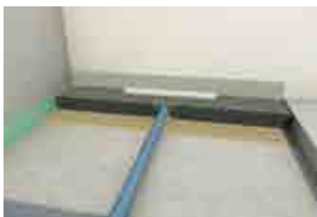
4. Connect the drain with pipe and make leak test
