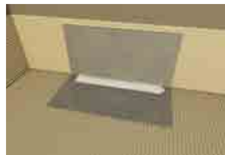
9. Set tiles up to the edge of the protection cover
