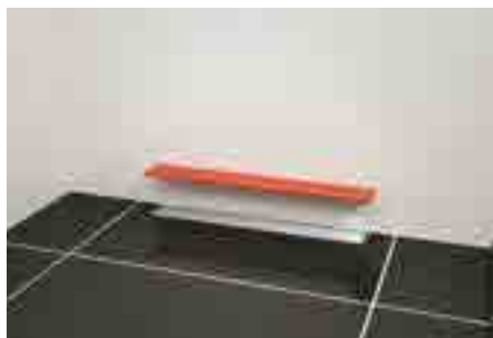
8. Set tiles, remove red protection cover.
