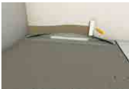
7. Apply liquid waterproofing on both sides of the sealing foil
