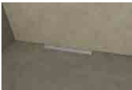
10. Remove protection cover and fill silicone into the surrounding gaps
