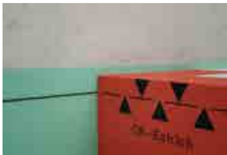
4. Take care, that the marks on the shower board are at the same level, than the floor screed will be.
