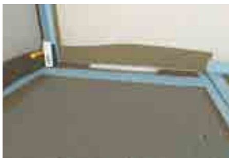
8. Attach sealing tapes, seal the entire shower area
