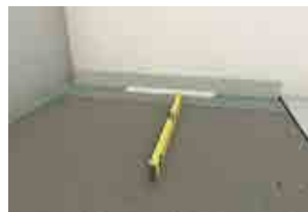
6. Insert screed with a minimum of 2% slope to the edge of the EPS-panel
