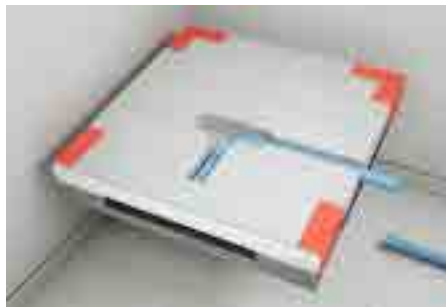
2. Turn shower board, define direction of the outlet pipe, remove EPS-supporting elements and insert pipe and fittings.
