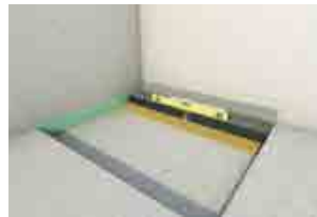
3. Position shower channel in the adhesive layer next to the wall. Check its horizontal position
