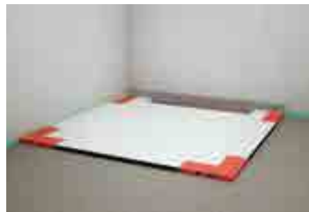
5. Floor screed level is proper with the marks „OK-Estrich“ on the board.
