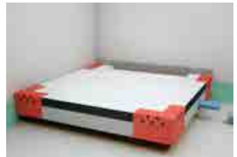
3. Turn again and set the shower board on e.g. tile glue, level it and connect to the pipe.
